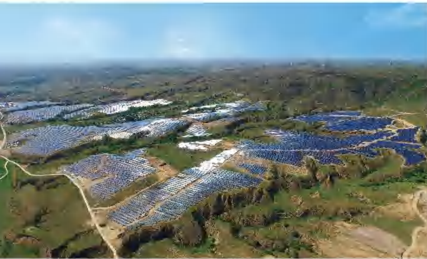
Shanxi Datong Photovoltaic Solar Power Plant Project
