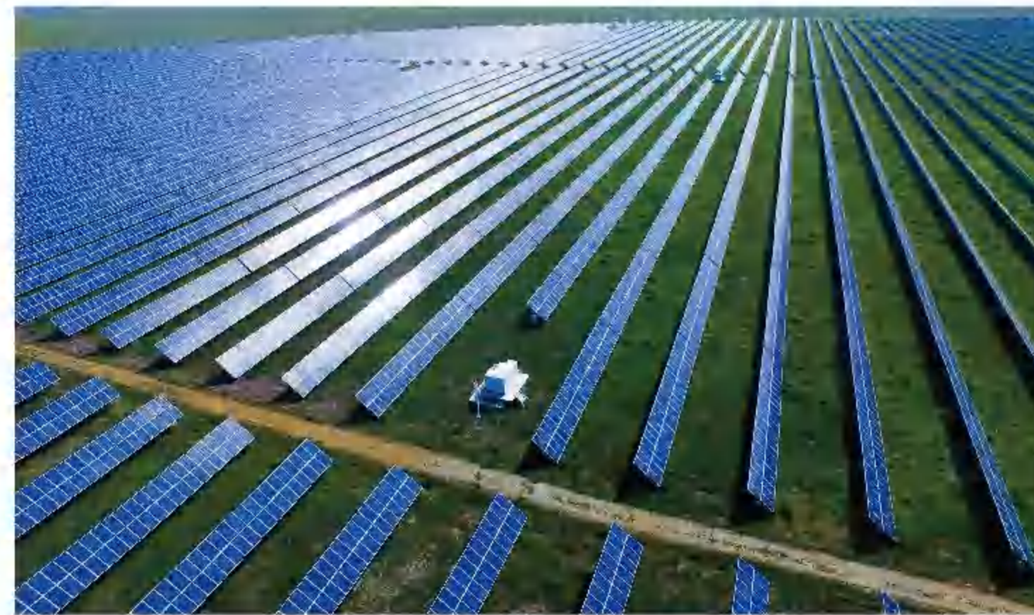
Hebei Zhangjiakou Photovoltaic Solar Power Plant Project
