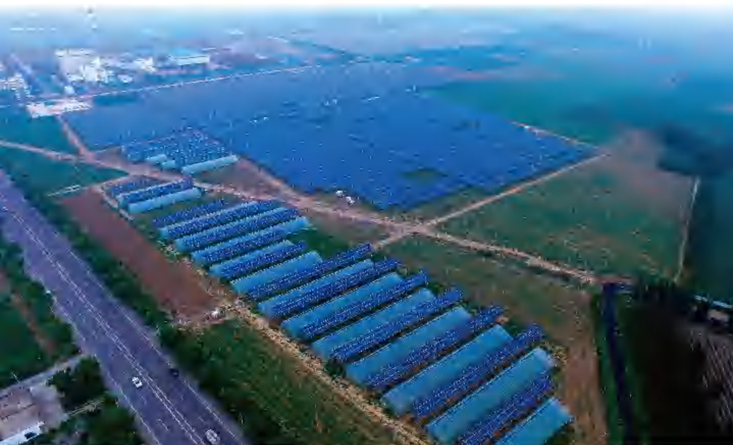
Shandong Tai'an Photovoltaic Solar Power Plant Project
